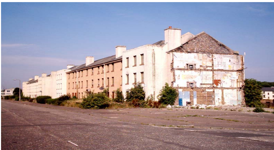
Traditional tenement housing, partially demolished. Photo: Adrian Welch www.edinburgharchitecture.co.uk
