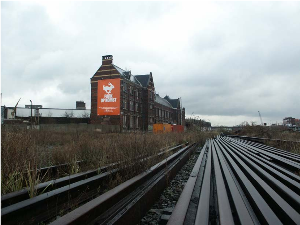
Derelict railway infrastructure in Spoor Noord, Photo: Planningscel, City of Antwerp
